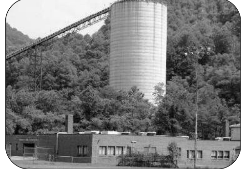
Massey's giant coal silo looms over Marsh Fork Elementary School, with a 2.8 billion gallon sludge pond lurking on the mountain above
