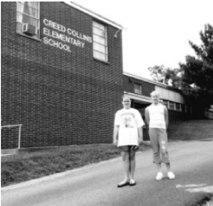
Betsy Nelson and Kelly Spangler stand in front of Creed Collins Elementary, one of five elementary schools in Ritchie County scheduled for closure under the county facilities plan. The community of Pennsboro has already lost a high school and a middle school.
